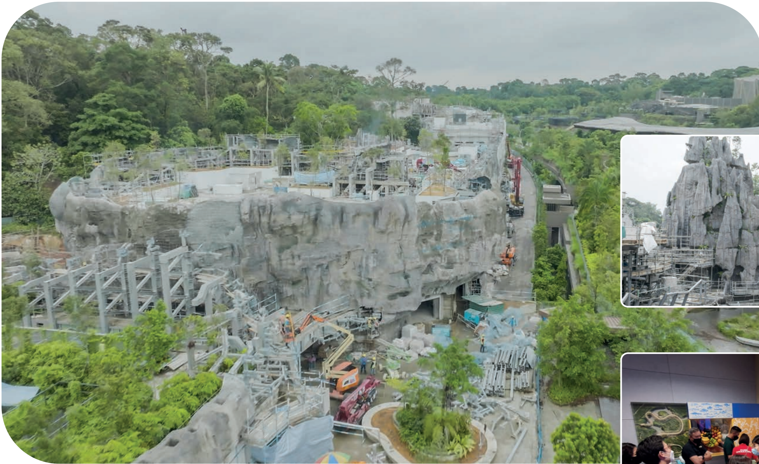
Construction progress is well underway for Rainforest Wild Asia.
